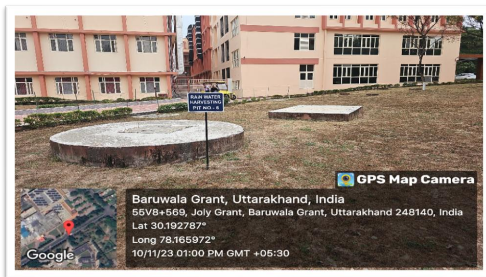
Rainwater harvesting pits with filter bed recharge near Cardiac OPD building
