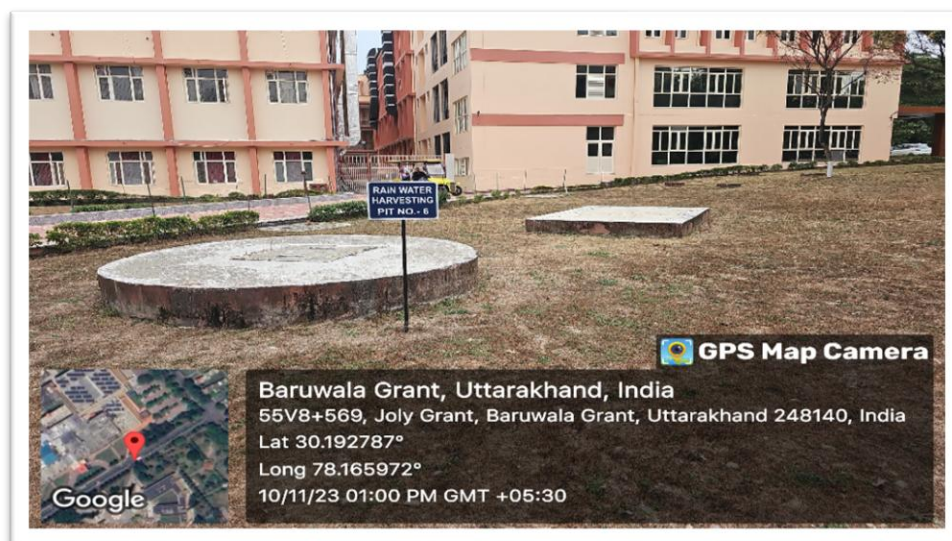
Rainwater harvesting pits with filter bed recharge near hospital building
